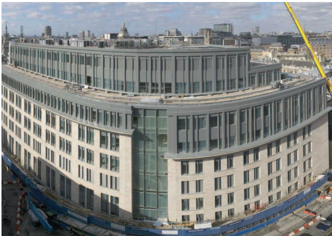
The new facility being built at St Bartholomew's Hospital in Farringdon.
